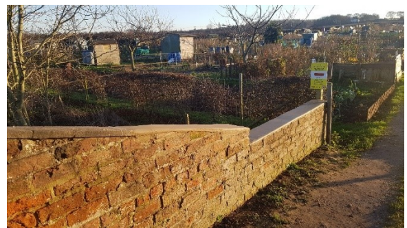
Allotment access bridge wall was re-topped just before Christmas 2019
